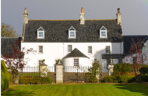
Uppat House with reinstated bowed roof.
