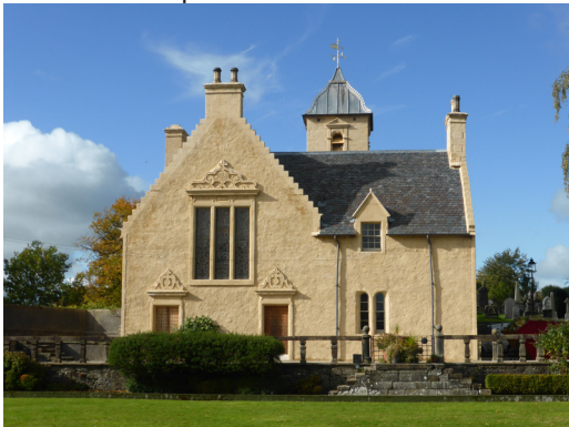
Cowane's Hospital with new limewash in its original tone.
