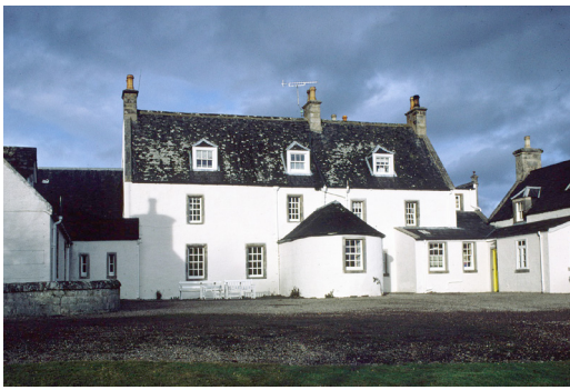
Uppat House before the fire which destroyed the roof.
