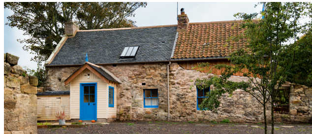
Grieve's House, Fountainhall, existing walls retained, jacked up and re-used in this conversion of redundant farm buildings.
